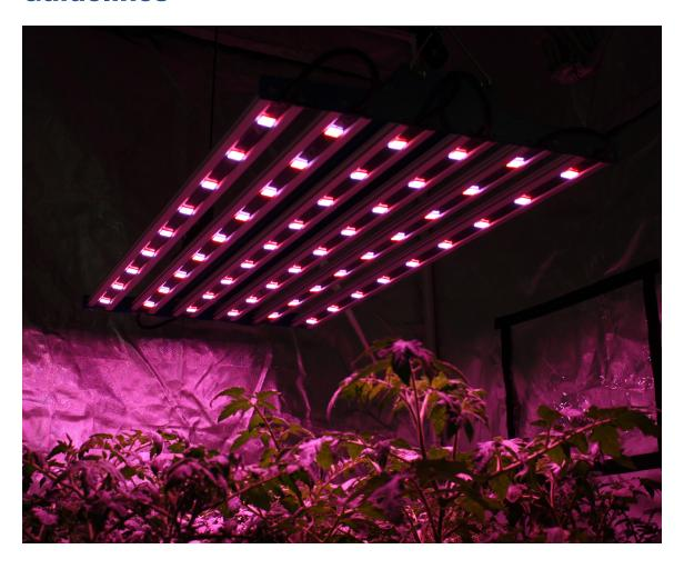
Using LED lights can require different mounting heights as compared to HID lighting. And while it's difficult to offer hard and fast rules for light mounting heights, we've come up with some general recommendations. If you're transitioning plants from legacy lighting sources to LED, you probably want to start on the high end of the scale of mounting heights listed below and gradually lower the fixture to increase intensity as your plants adapt to their new lighting source.
